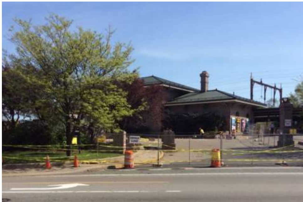
CONTRUCTION AT MORRISTOWN TRAIN STATION – MAY 12, 2016
