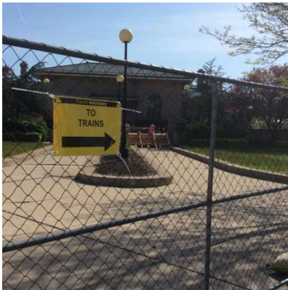
CONTRUCTION AT MORRISTOWN TRAIN STATION – MAY 12, 2016
